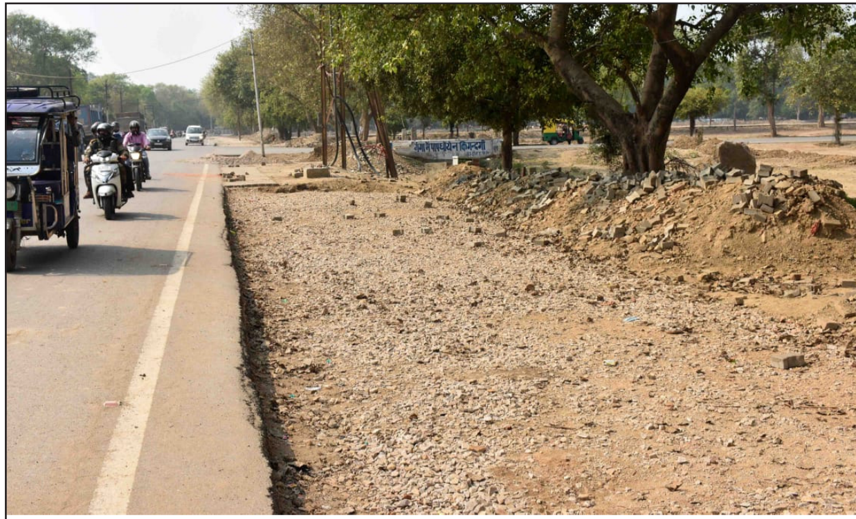
The road is being widened at the parade ground
